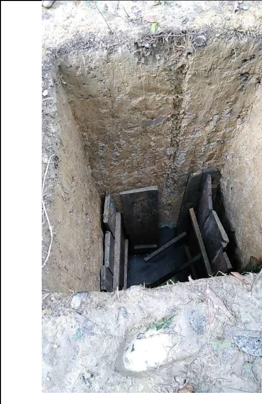
Pit showing wooden safety boarding
