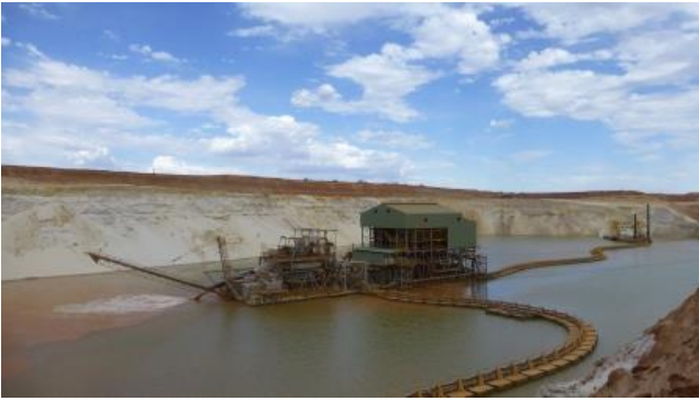
Dredging at Cristal Mining's Ginkgo Mine (Source: Earth Science Australia).
